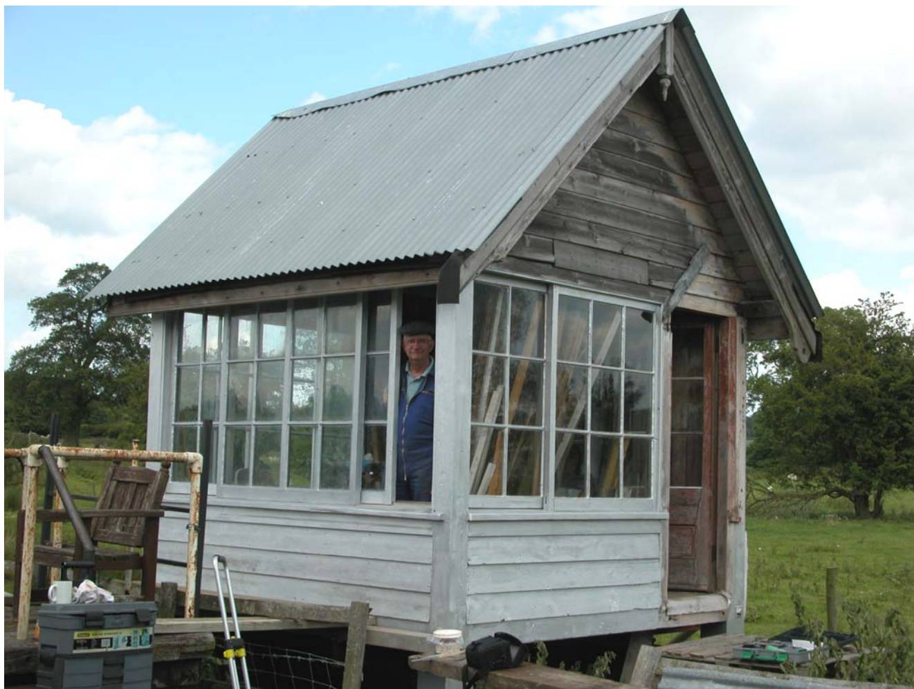
All the windows have now been restored and replaced into the Waterhouse Signal Box
