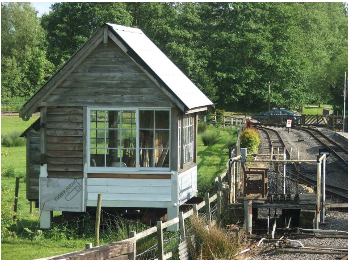
The restored sashes have been replaced in the Leek and Manifold Waterhouses Signal Box
